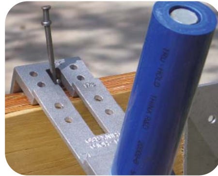
6 Place Tru-Hold® on the form with the identification layout* located on the center of elongated layout opening
