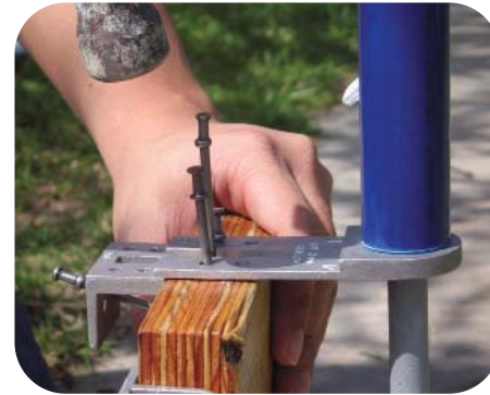
7 Nail down Tru-Hold® on the form by following the stop and step face for different size of form (2x4 or 2x6 lumber)
